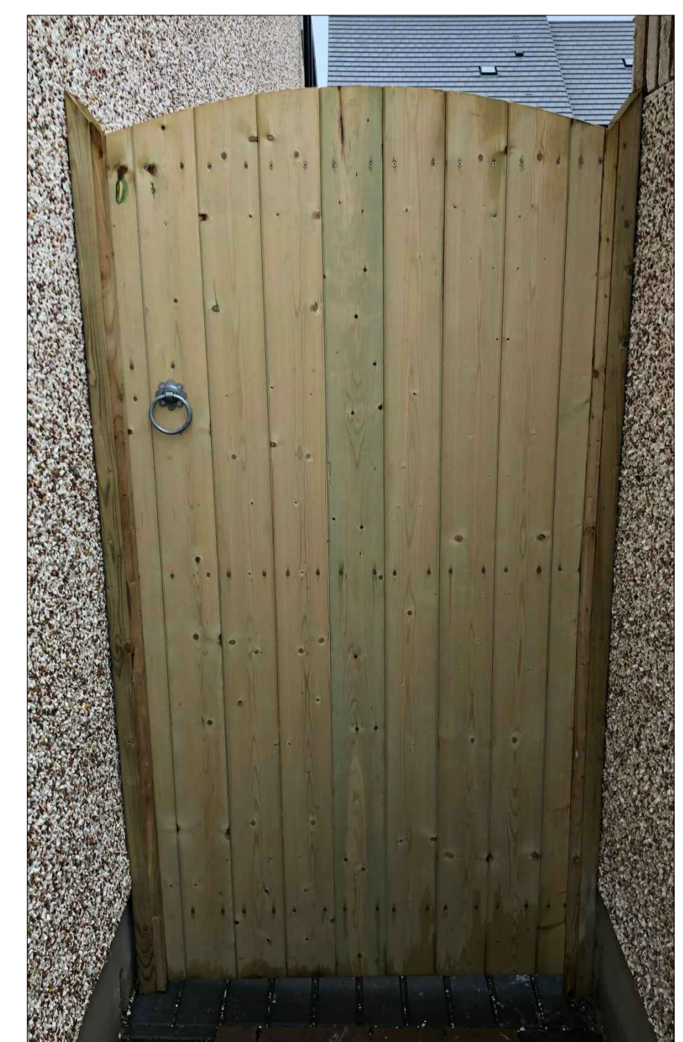
1800x850mm Wooden side door fixed to concrete 'H' post.
